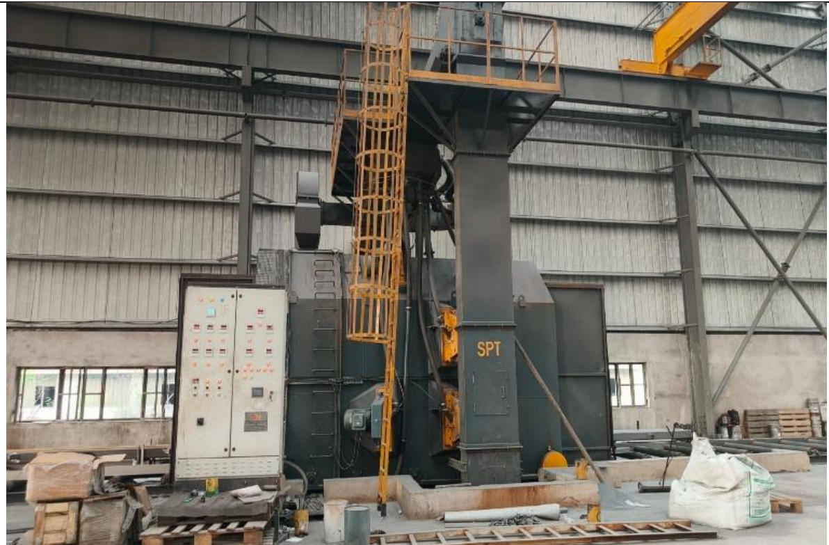
SHOT BLASTING/GRIT BLASTING
